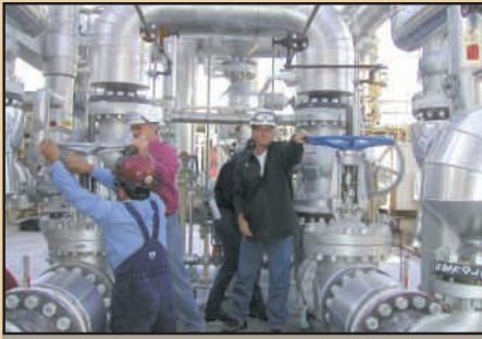
Installation of the first commercial IsoTherming™ unit.
